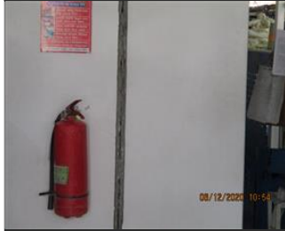
Photo of fire safety equipment Fire extinguisher.JPG
