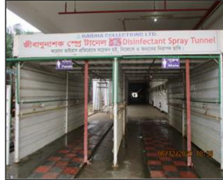
Photo of the inside of the main production hall Covid 19 prevention measure Disinfectant chamber.JPG
