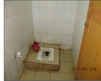
Photo of the sanitary facilities Toilet area.JPG
